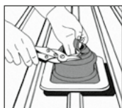
1. Adjust DEKTITE® to the pipe.
